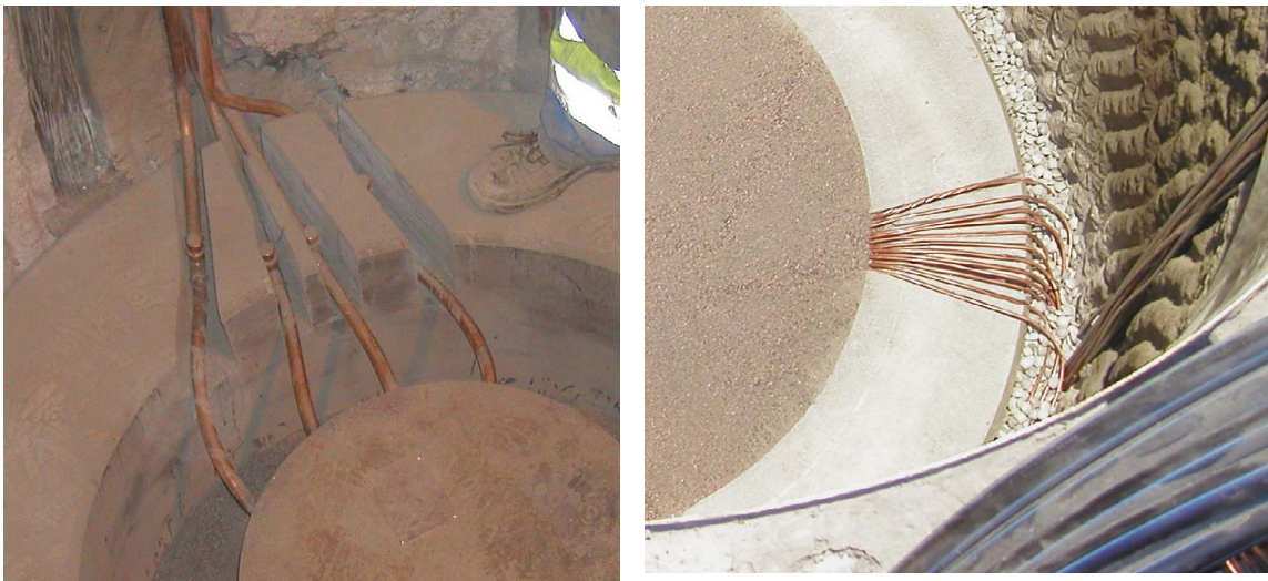
Figure 5-7. Possible pathways for leakage from sand shield. Left: Slots for heater power cables. These were subsequently sealed with bentonite powder. Right: External thermocouples from heater.
